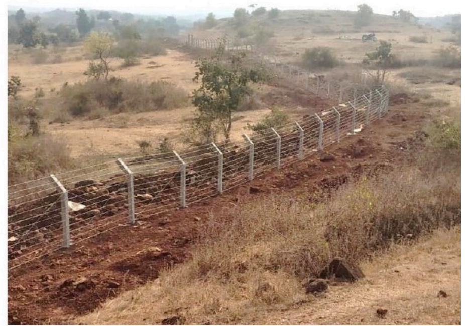
Fencing work at the acquired site
