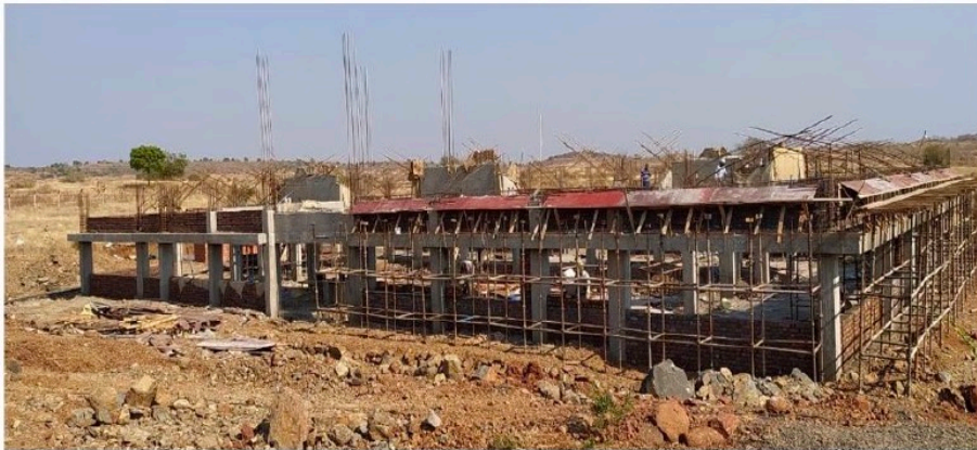
RCC Works for construction Site office
